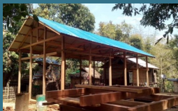
Church building Construction.
